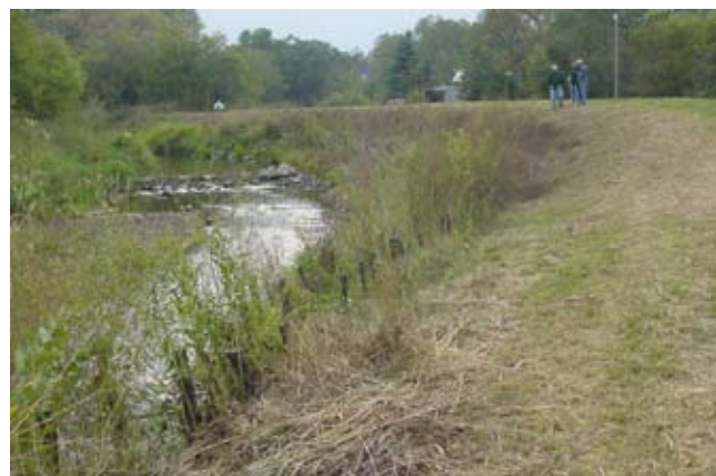
Figure TS14I-22 Live pole cuttings after one season
