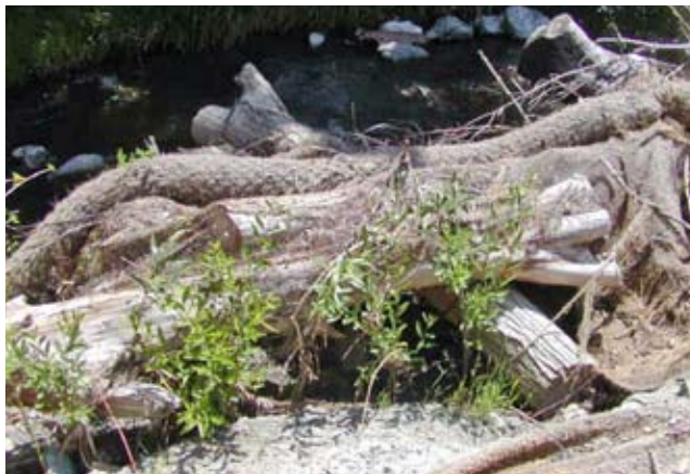
Figure CS15-4 Evidence of scour and exposure of the log structures
