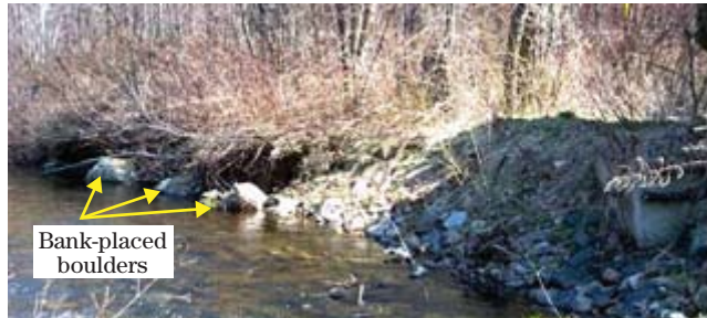
Figure CS8–21 Site 2—looking downstream at bank-placed boulders, station 2+40
