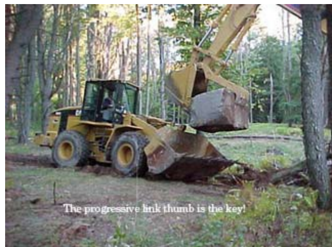
Figure CS6–10 Loading a typical wall rock used for vane construction
