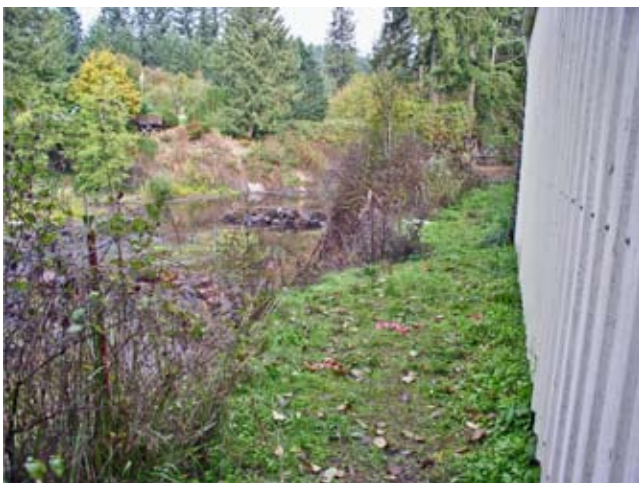
Figure CS18–9 Looking upstream at the project bank. Less than 5 feet of bank remained from the building to the edge.
