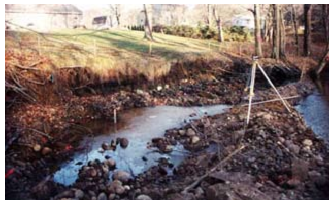
Figure CS8-18 Site 7 during construction—looking downstream at station 14+25
