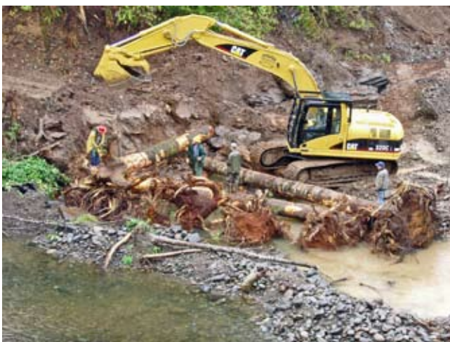
Figure CS18–14 (a) Construction of the upstream ELJ. A temporary cofferdam was placed to dewater the construction area; (b) construction of one of the project stream barbs. Photo is taken looking up the axis of the barb structure.
