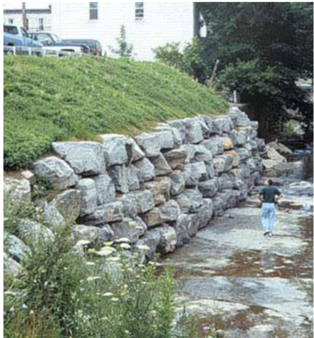
Figure CS4-13 Completed wall
