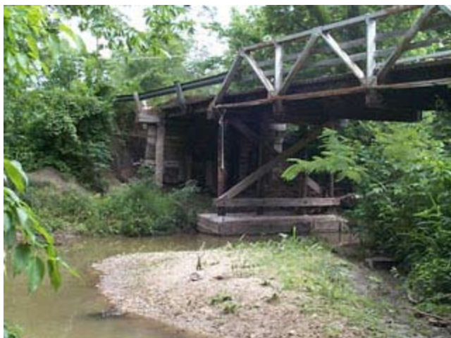
Figure CS2-1 Original timber-plank bridge structure
