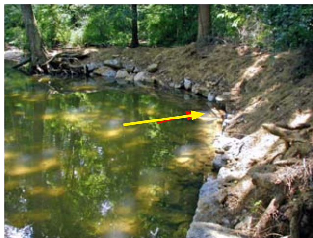
Figure TS140–1 (a) LUNKERS being installed as part of a bank stabilization project; (b) Completed LUNKERS project; LUNKERS are under the stone (Photo courtesy of Mike Martyn, USACE)
