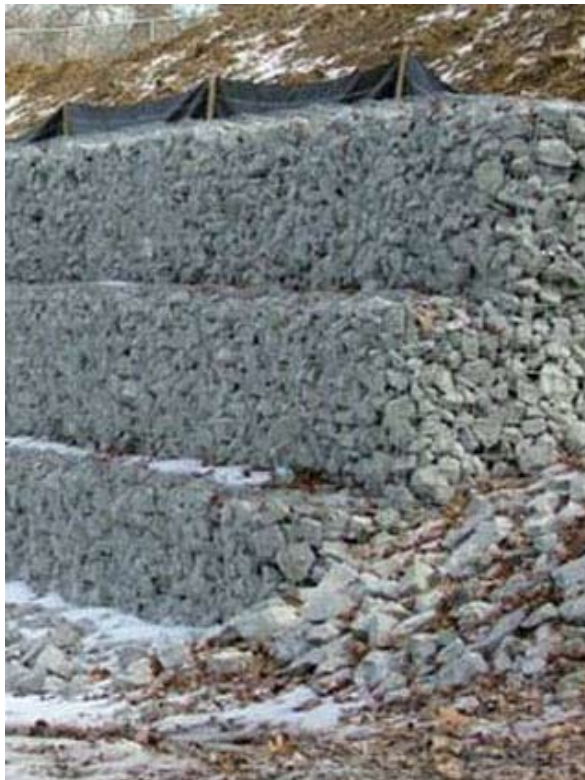
Figure CS4-3 Bin wall
