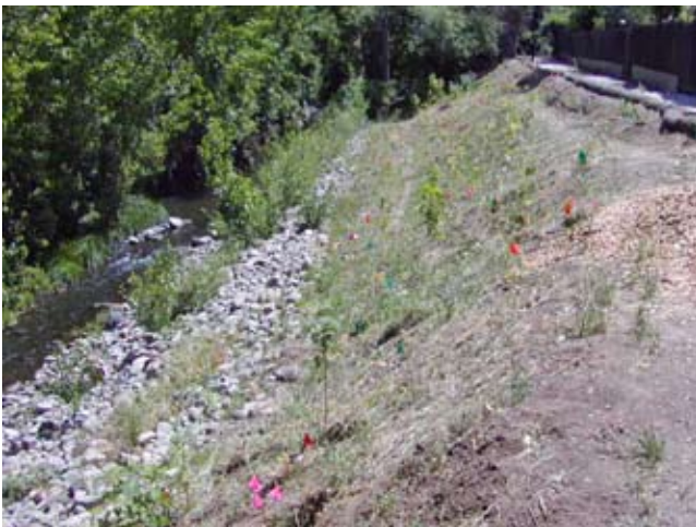
Figure CS15-12 Revegetated slope 1 year later
