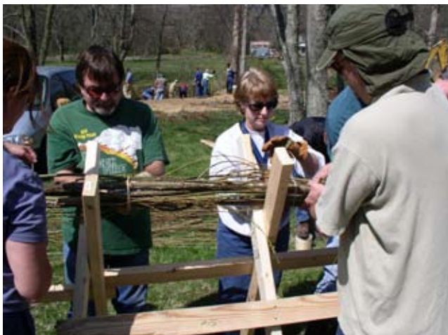
Figure TS14I-18 Assembling fascines
