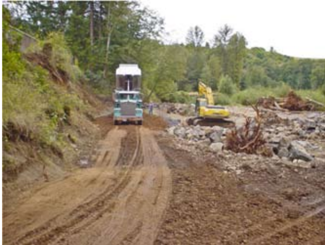
Figure CS18-17 (a) Access road was constructed to allow haul trucks to drive onto each lift, dump fill material, and provide compaction; (b) fill material was spread uniformly with a dozer.
