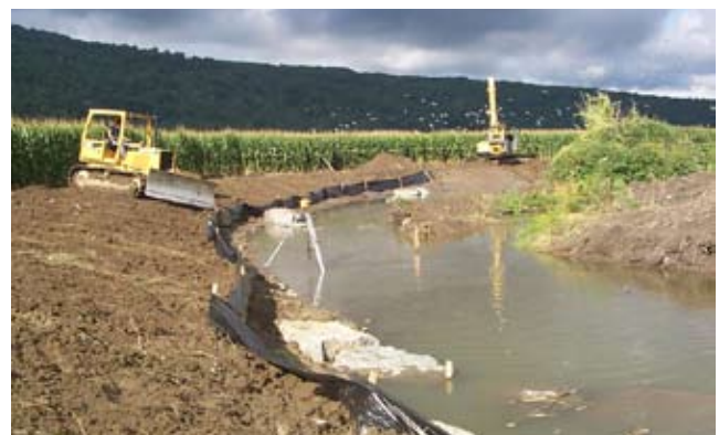
Figure CS7-5 J-hook vane installed and final grading of streambank followed by seeding and mulch, Spafford Creek, NY
