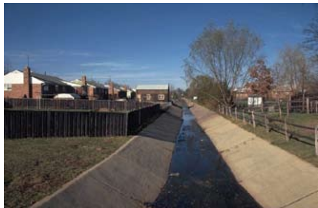
Figure 4-3 Lined channels may be necessary, based on boundary constraints, drainage needs (discharge capacity), and maintenance costs.
