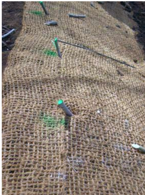
Figure TS14I-39 Live cuttings installed in fabric
