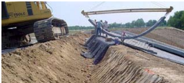
Figure TS14L-20 ACB termination trench
