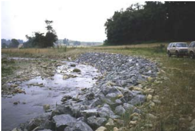
Figure CS5-6 Upper riprap, July 1998, 3 months after construction
