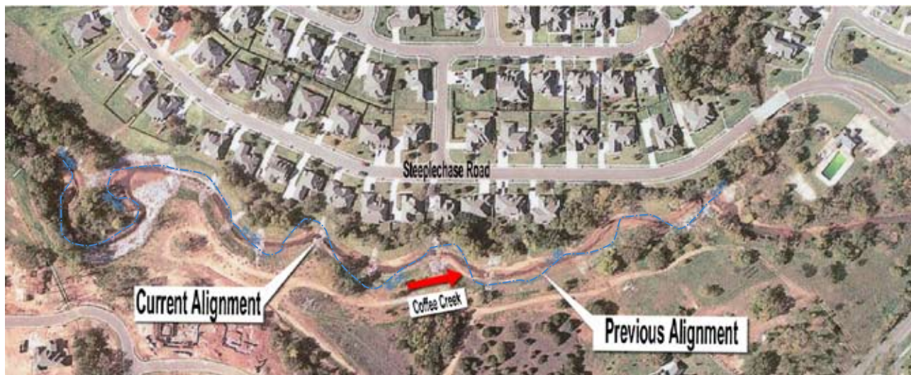
Figure CS16-6 Aerial view of project channel alignments
