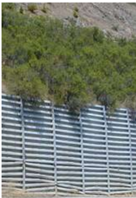
Figure CS4-3 Bin wall
