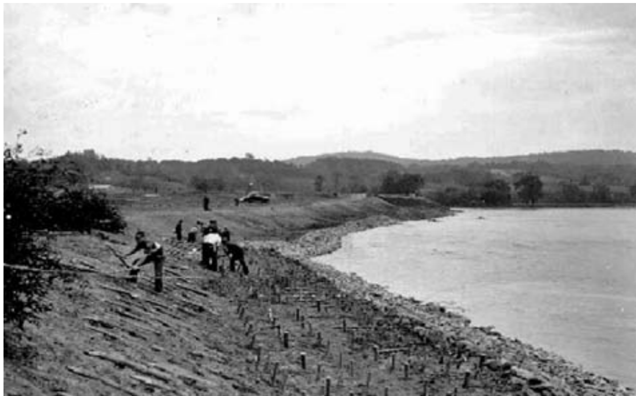
Figure E-1 Workers installing live willow stakes and brush matting on a terraced streambank, Winooski River, VT (September 1938)
