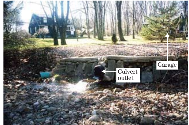
Figure CS8-14 Site 5 before project—looking at head-wall at station 11+10
