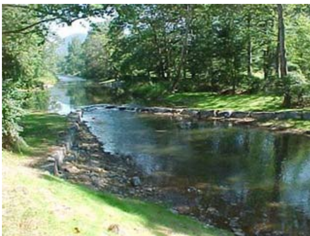
Figure CS6–17 Cross vane illustrating the proper upstream fill along the vanes, leaving a flat horizontal ramp along the vane
