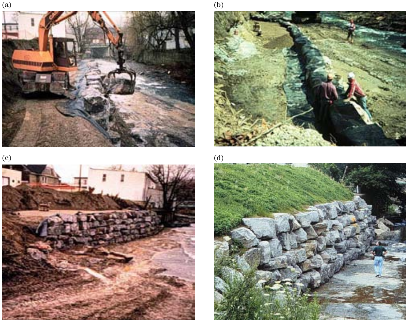
Figure TS14A-16 Construction of a geotextile reinforced slope with large derrick stone armoring at toe of slope
