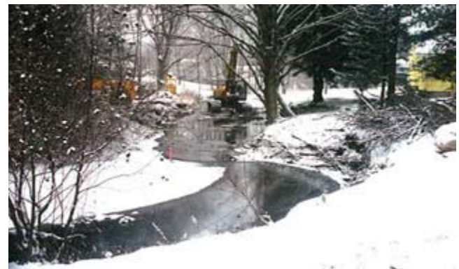
Figure CS8-16 Site 6 during construction—looking downstream at station 12+00
