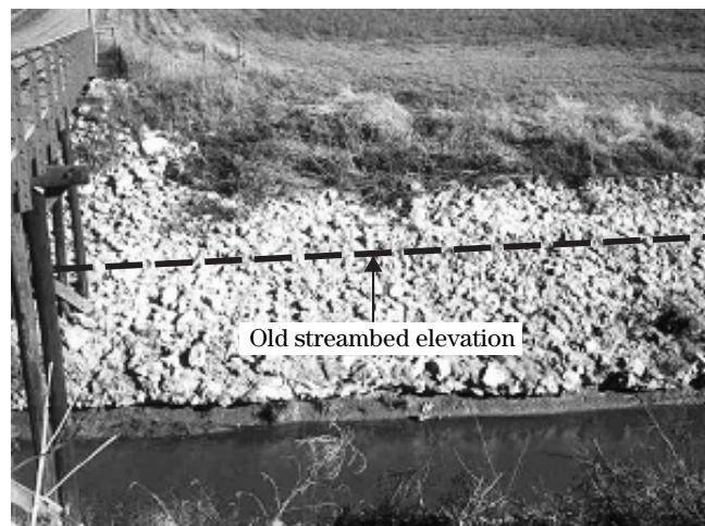
Figure TS3B-4 An NRCS bank stabilization site that did not include streambed stabilization, (Page County, IA)
