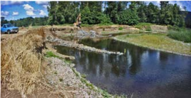
Figure CS17–7 Looking downstream at initial installation of two barbs before bank shaping, during low summer flows (Photo courtesy of Scott Wright)
