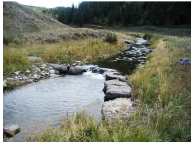
Figure TS14G-9 A J-hook grade control structure
