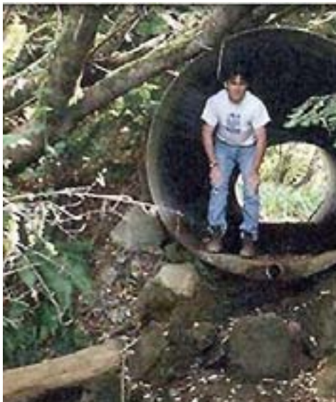
Figure TS14N-18 A significantly perched culvert ( Photo courtesy of Dick Quinn, USFWS, Newton, MA )
