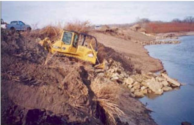
Figure CS9-6 Building weir on site 28
