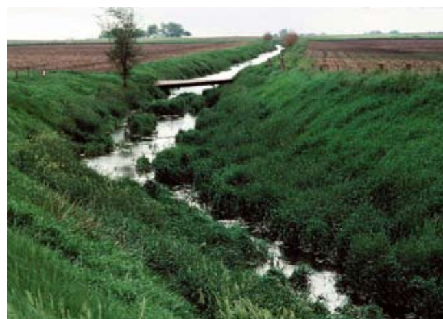
Figure 10-2 Drainage ditch constructed in north-central IA
