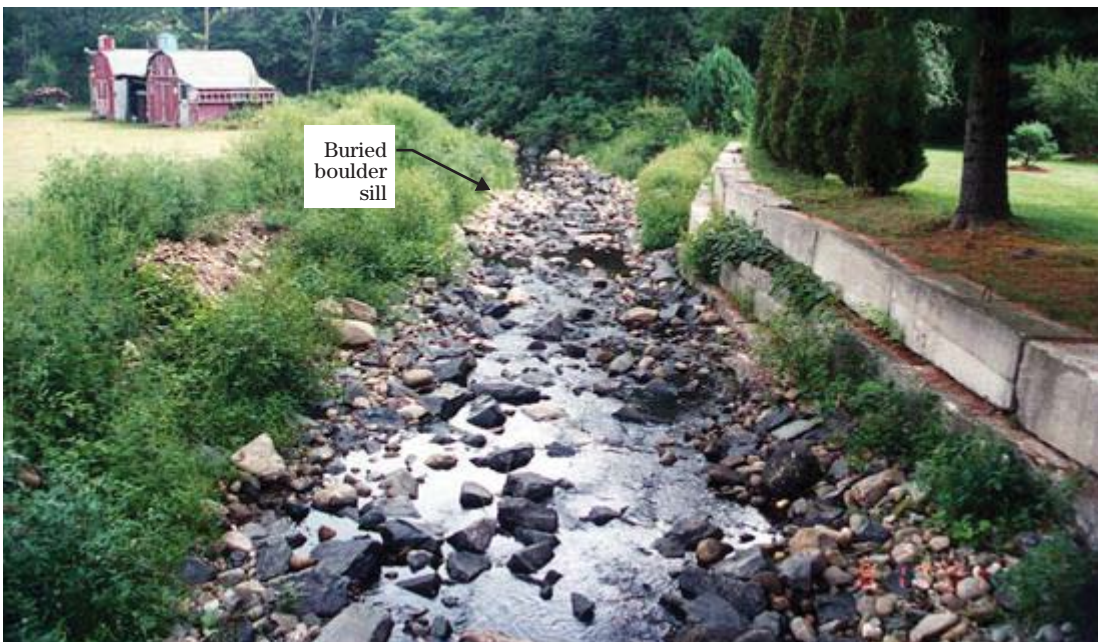
Figure CS8-12 Site 1 after project—looking downstream from Prospect Street Bridge
