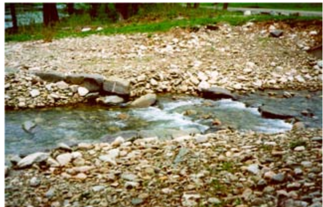
Figure CS6–16 Tip-out due to scour from a suck hole
