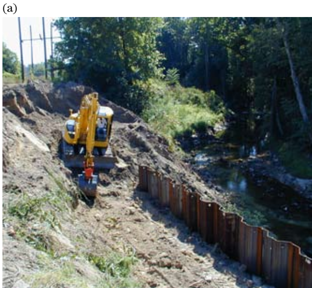
Figure TS14A-11 Sheet pile wall at toe of slope in Tarboro, NC. Vegetation will be established above wall. Note erosion control fabric.
