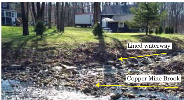
Figure CS8-15 Site 5 after project—looking at lined waterway, station 11+10
