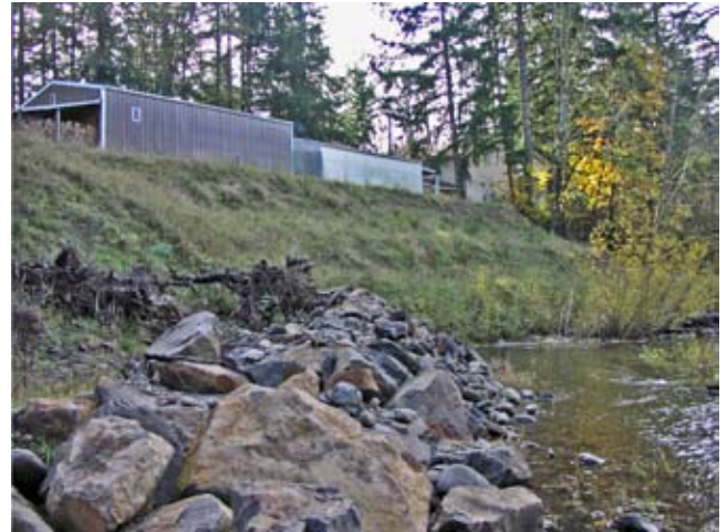
Figure CS18-2 Completed reinforced earth embankment, stream barb, and bank vegetation 1 year following construction
