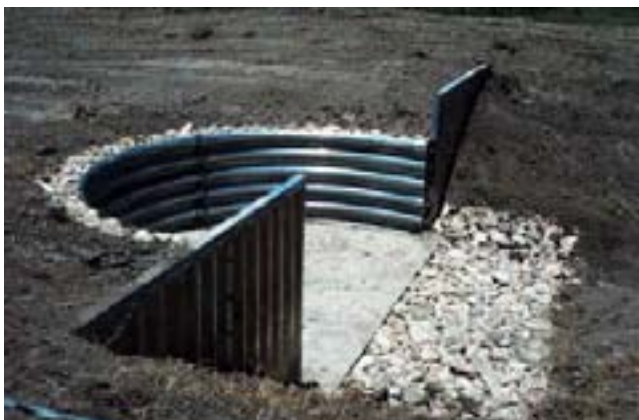
Figure TS14P-29 Grade stabilization structure
