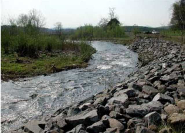
Figure CS5-8 Upper riprap, April 2003
