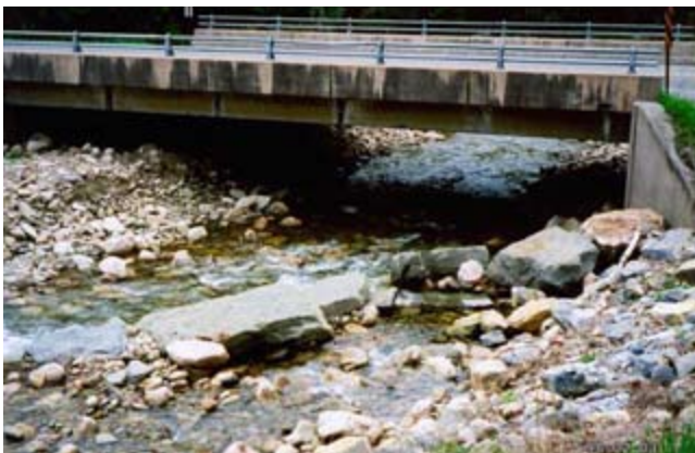
Figure CS6–15 Vane with a tip-out vane rock due to the scour from a gap hole
