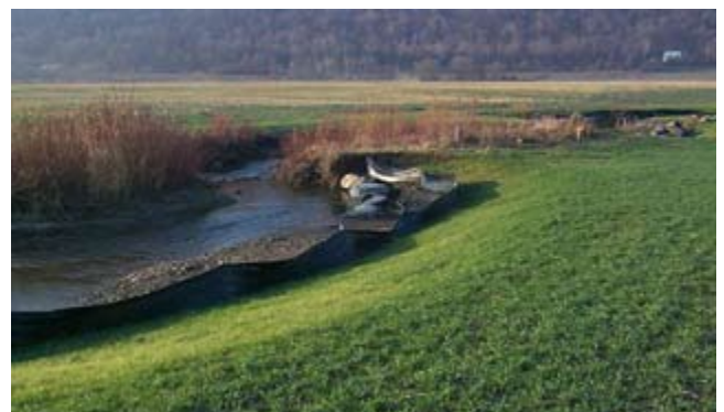
Figure CS7-7 Completed section of streambank stabilization to include J-hook vane and intentional point bar, Spafford Creek, NY
