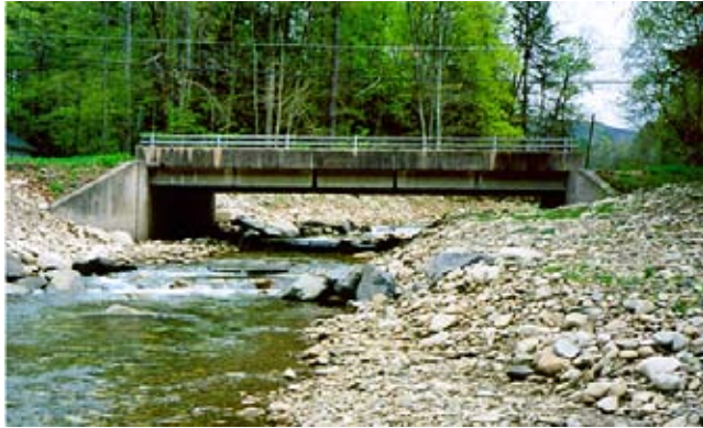
Figure CS4-4 Concrete wall alternative
