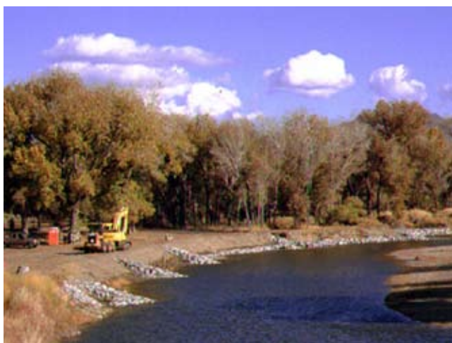
Figure TS14A-10 Barb structures installed to protect toe of slope from erosion
