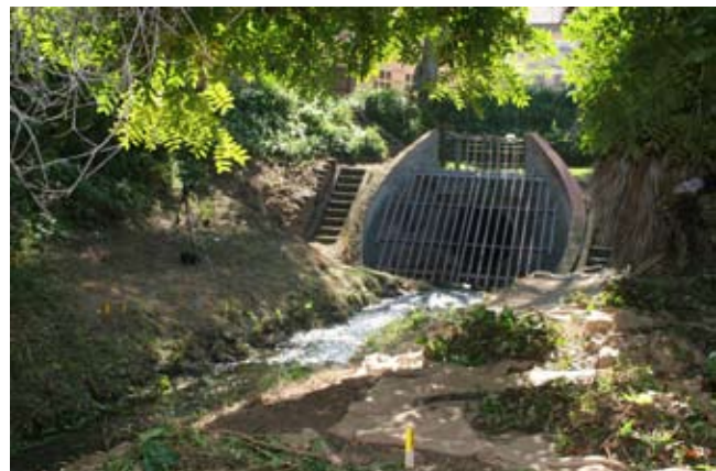
Figure 2–3 Daylighting stream project
