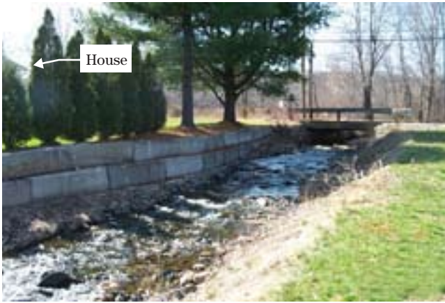
Figure CS8-11 Site 1 after project—looking upstream at Prospect Street Bridge
