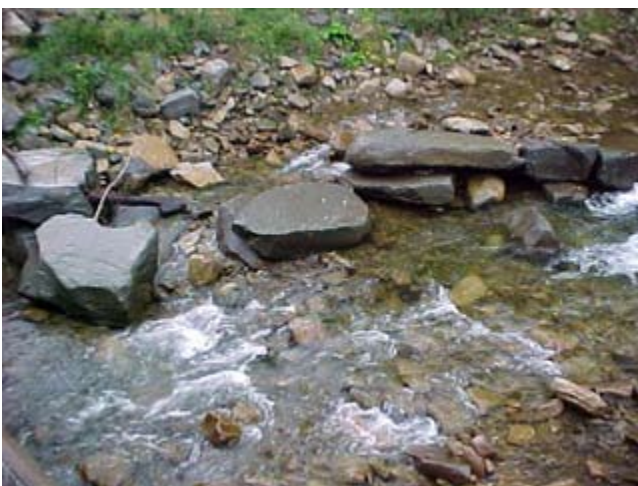
Figure CS6-12 Example of vane rocks with small footer rocks and inadequate long-term performance
