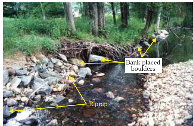
Figure CS8-20 Site 7—looking downstream at bank-placed boulders, station 14+50
