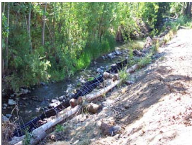
Figure CS15-5 Live siltation installation
