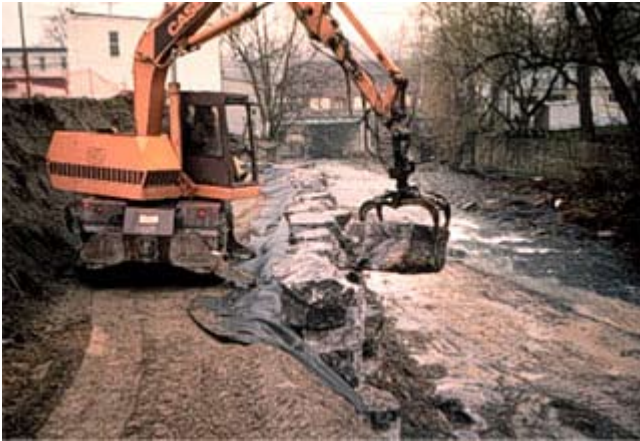
Figure CS4-10 Stacked riprap face placement
