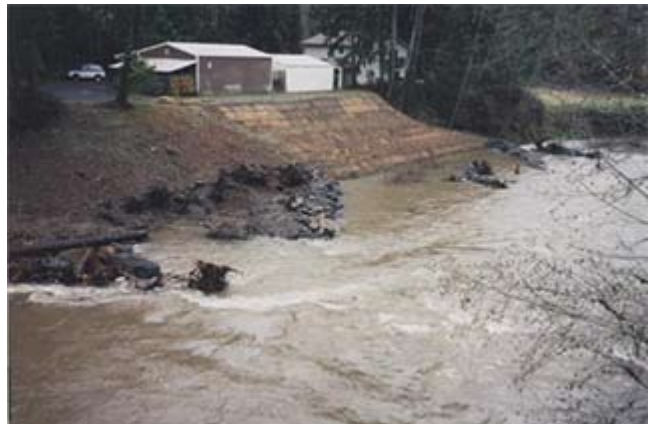
Figure CS18–22 (a) Project nearing completion. All primary project components are complete except for embankment vegetation. (b) November 2004 flooding approximately 2 months after the completion of construction. Note high velocities deflected at the upstream log jam (on left of photo) and the subcritical, low-shear stress flow condition in the near bank region along the embankment toe.
