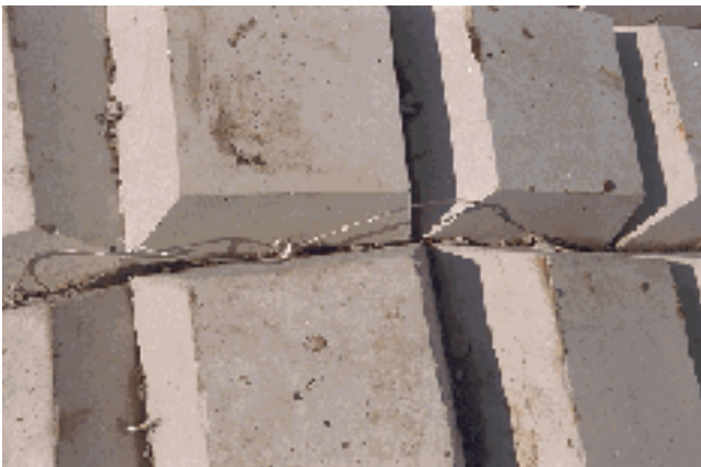
Figure TS14L-8 Steel cables
