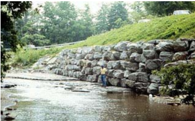
Figure CS4-12 Completed wall
