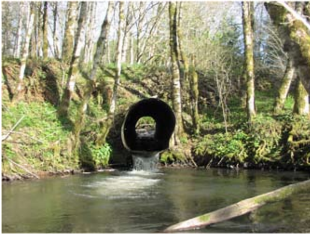
Figure TS14Q-3 Forest road culvert acting as fish passage barrier (Photo courtesy of Christi Fisher)
