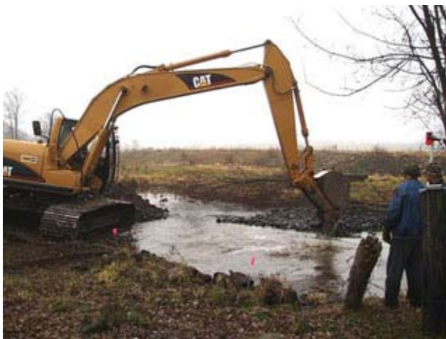
Figure CS3-5 Removal of rock dam crossing, Nov. 2001
