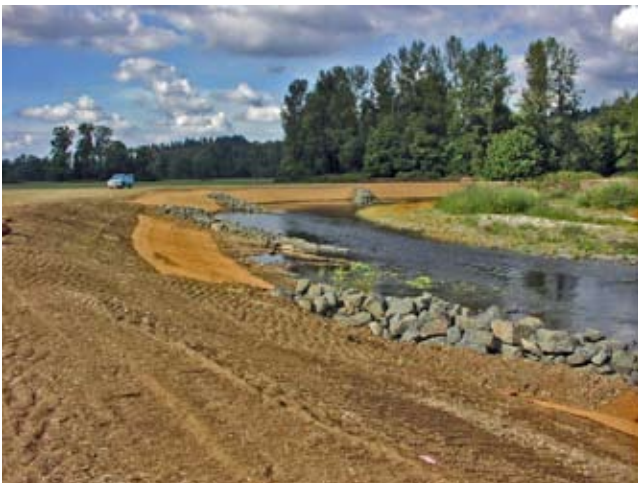
Figure CS17–9 Looking downstream at completed project showing barbs and erosion control mat during summer flow ( Photo courtesy of Scott Wright )
