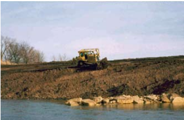
Figure CS9-8 Bank shaping with bulldozer
