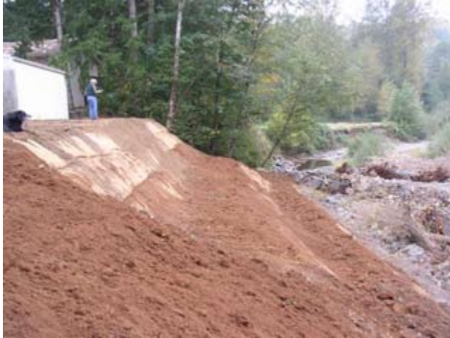
Figure CS18–23 (a) Looking downstream along the embankment immediately after construction and before planting of vegetation (August 2004); (b) Same view of project in December 2005 showing vegetation establishment. Note location of buildings in both photos.
