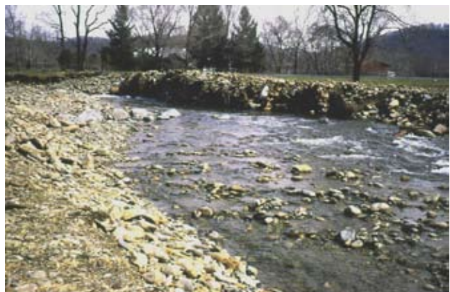
Figure CS5-5 Upper rootwads after construction, July 1998
