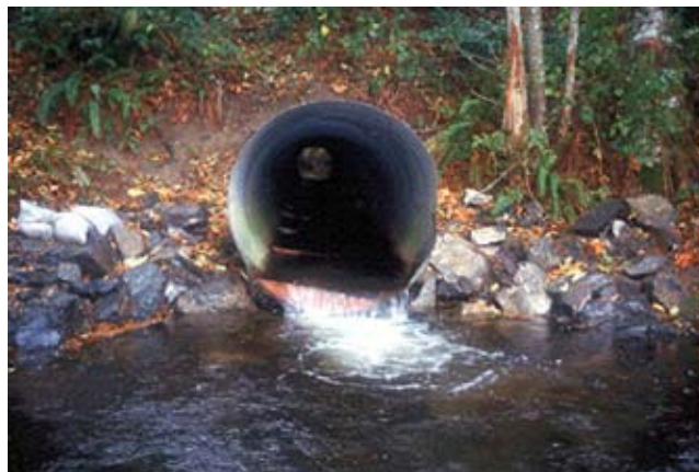
Figure TS14N–21 Round, corrugated metal culvert retrofitted with corner baffles to improve fish passage
