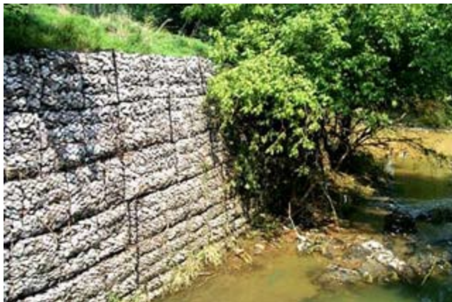
Figure TS14A-12 Gabion wall constructed at toe of slope enabled reconstruction of failed slope where right-of-way limitations prevented flattening of the upper slope and use of other conventional toe protection measures at the toe
