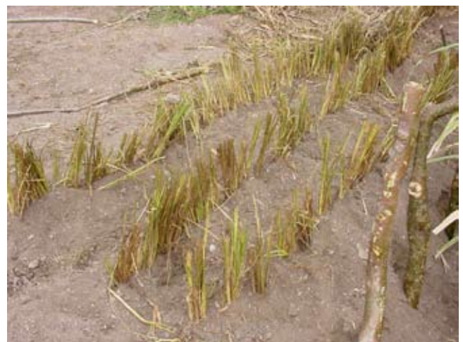
Figure TS14I-37 Crimped straw
