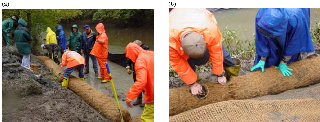
Figure TS14I-8 Installation of coir fascines: (a) Anchoring; (b) Tying of the coir fascines together ( Photos courtesy of Robin B. Sotir & Associates, Inc. )
