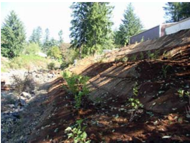
Figure CS18–24 (a) Looking upstream along the embankment immediately following placement of vegetation (August 2004); (b) Same view of project in December 2005 showing establishment of vegetation with vigorous willow growth along the embankment toe. Note location of buildings in both photos.
