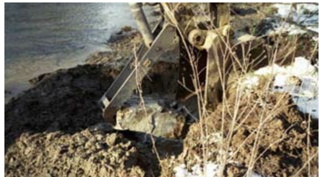
Figure CS6-13 Setting a footer rock (upstream direction is to the right)
