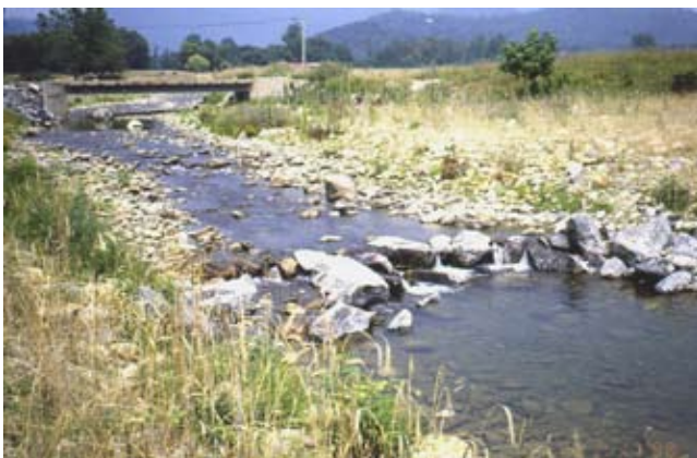
Figure CS5-4 Weir #7, July 1998
