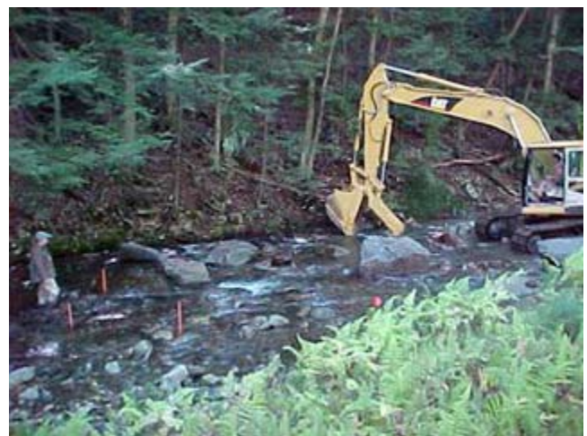
Figure CS6-9 Staking out a cross vane
