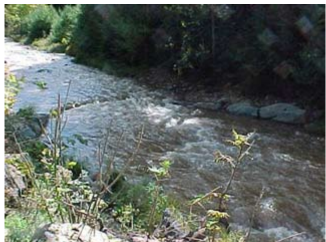
Figure CS6-8 Cross vane on Big Bear Creek
