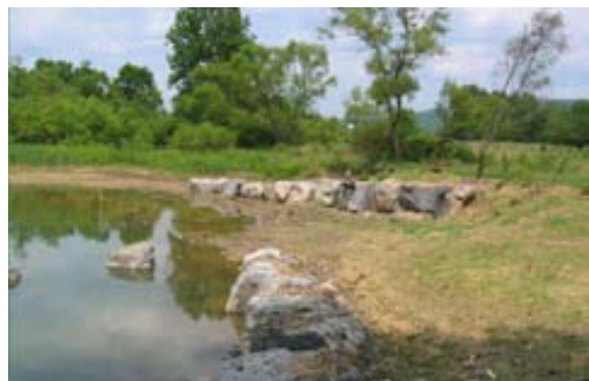
Figure TS14H-6 Rock vane
