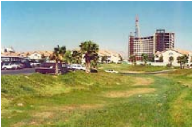
Figure 7-2 Grass-lined threshold channel
