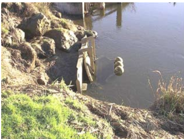
Figure TS14N-28 Self-regulating tide gate
