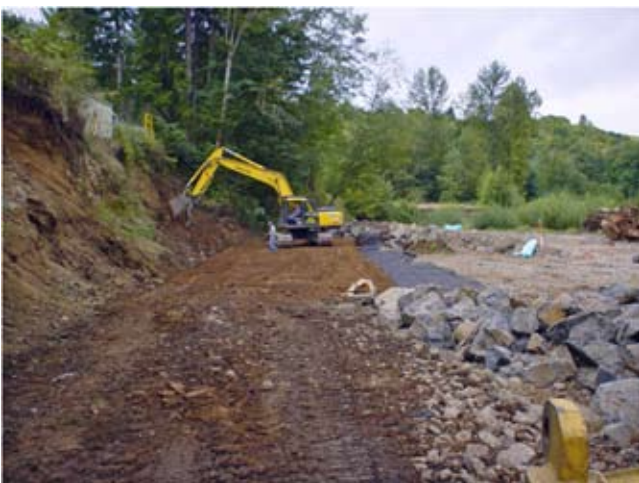
Figure CS18-18 (a) First soil lift on top of the base foundation geogrid. Portion of upstream stream barb is in foreground, and downstream barb is seen in distance. Geogrid extending from the soil is wrapped over to encapsulate the lift after compaction and grade have met specification; (b) Grade was checked at multiple locations on each soil lift. Base course geogrid can be seen underlying fill material.
