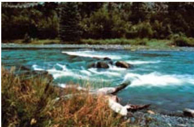
Figure 11-33 W-weir installed on the Uncompahgre River, CO
