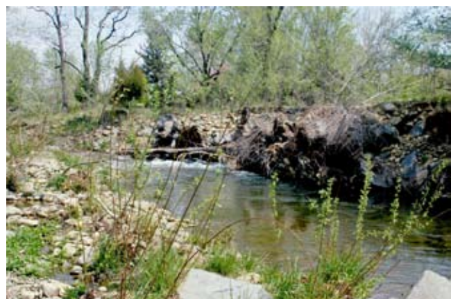
Figure CS5-16 Upper rootwads, April 2004, after Hurricane Isabel
