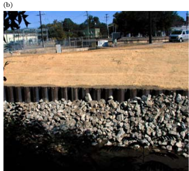
Figure TS14A-11 Sheet pile wall at toe of slope in Tarboro, NC. Vegetation will be established above wall. Note erosion control fabric.
