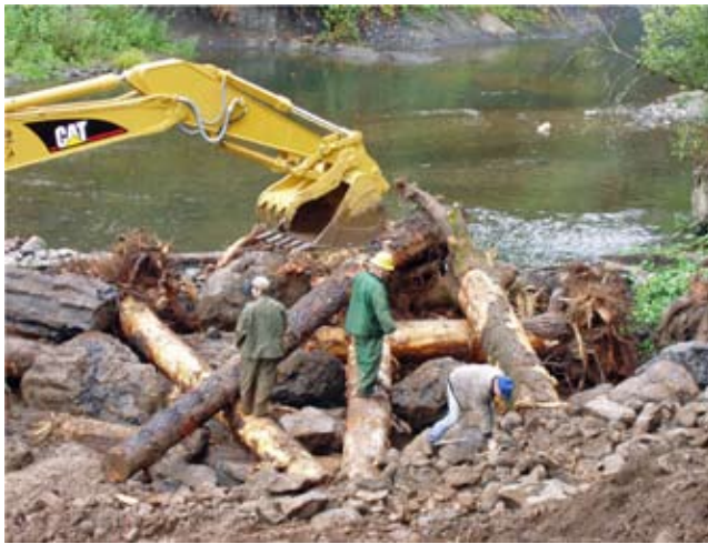
Figure CS18-21 (a) Excavator used a chain to place log members in position for the construction of the engineered log jams. Individual log members were bolted together, and rock ballast was placed. Note pool in background. (b) The presence of salmon in the immediate vicinity of the construction area required careful management of turbidity and site runoff. Photo was taken at the pool noted in figure CS18-21a.
