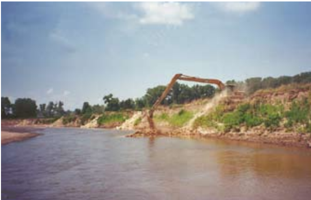
Figure CS9-7 Weir construction on site 22
