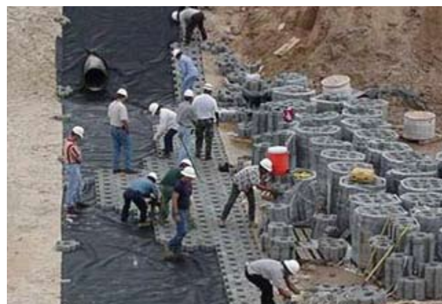
Figure TS14L-19 Hand placement of ACB blocks
