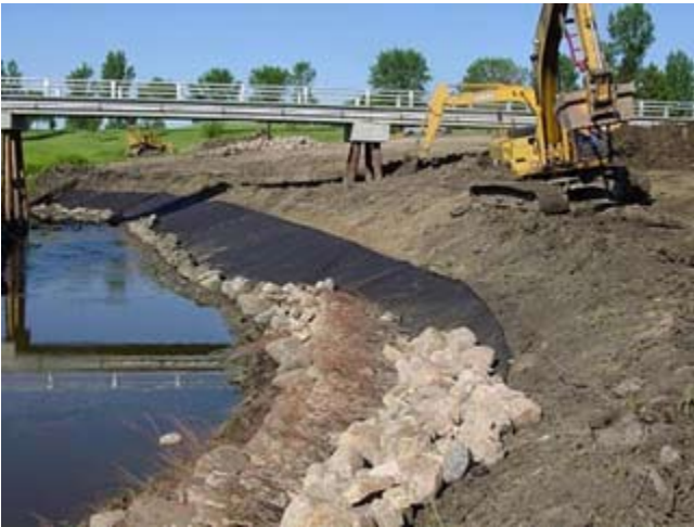
Figure CS11–17 Rock toe being placed over geotextile. A layer of live willow branches is visible within the rock toe.
