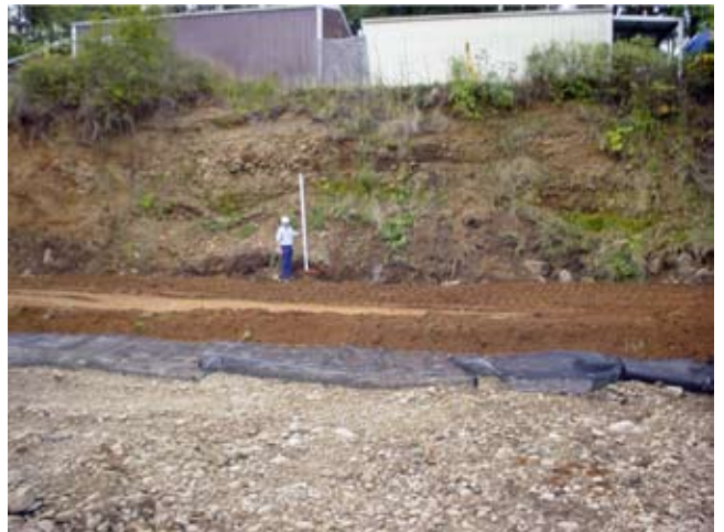
Figure CS18-18 (a) First soil lift on top of the base foundation geogrid. Portion of upstream stream barb is in foreground, and downstream barb is seen in distance. Geogrid extending from the soil is wrapped over to encapsulate the lift after compaction and grade have met specification; (b) Grade was checked at multiple locations on each soil lift. Base course geogrid can be seen underlying fill material.
