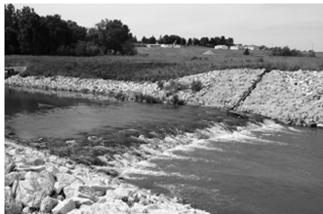
Figure TS3B-5 HCA steel sheet pile weir with riprap and cement grout that protects a large sewer main for the City of Denison, IA
