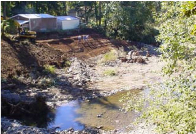
Figure CS18–22 (a) Project nearing completion. All primary project components are complete except for embankment vegetation. (b) November 2004 flooding approximately 2 months after the completion of construction. Note high velocities deflected at the upstream log jam (on left of photo) and the subcritical, low-shear stress flow condition in the near bank region along the embankment toe.
