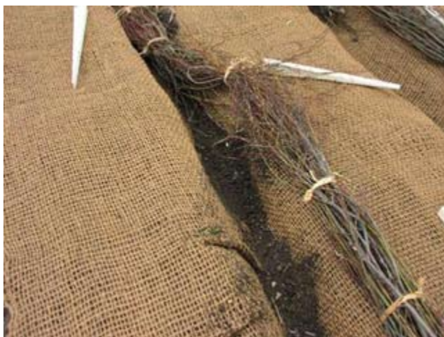
Figure TS14I-40 Combining fascines and fabric
