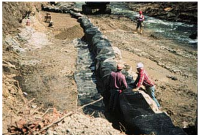
Figure CS4-9 Primary geotextile anchorage length
