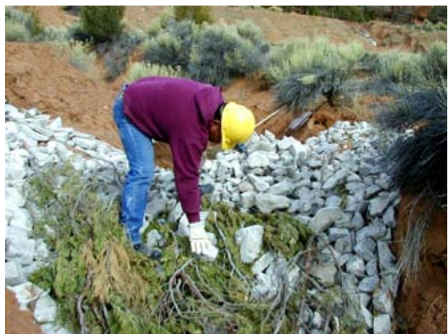
Figure TS14P-24 Rock and brush dam under construction in AZ (Photo courtesy of Pete Bautista)
